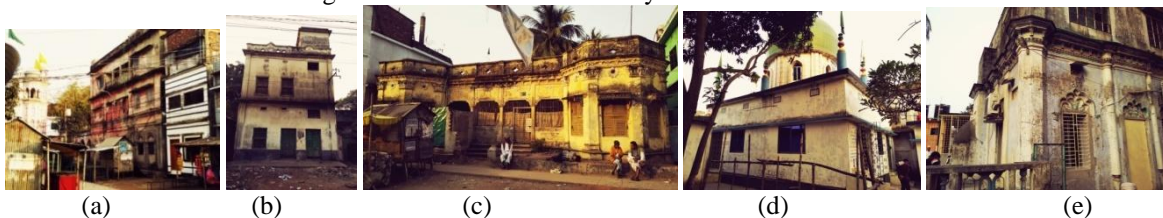
Figure 3. (a) Colonial House : : Chowdhury House (b) Colonial House : : Chairman House (c) Colonial House : : Sardar House (d) Colonial Architecture : : Kiamuddi Shah Tomb (e) Colonial Architecture : : Boro Bari Mosque
